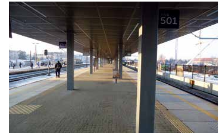
Railway stations Železničke stanice
